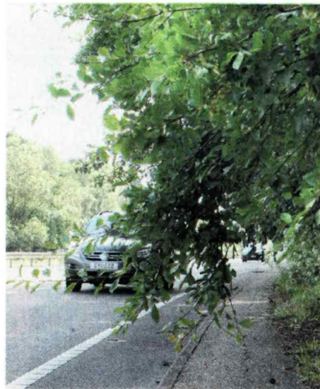
Hedgerow overgrowing the highway on the A24.
