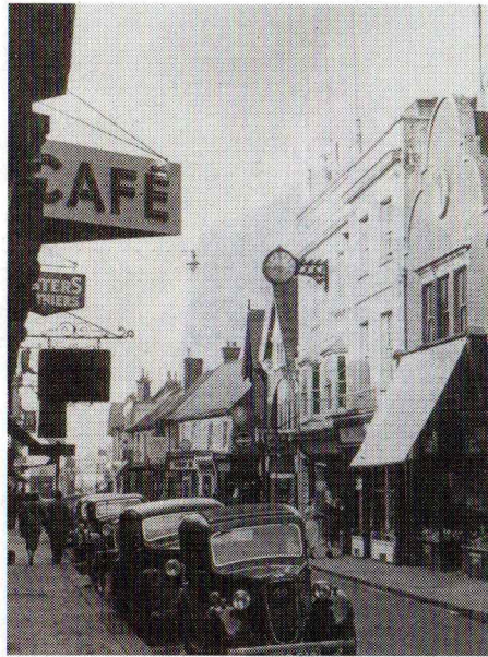
Rooflines are always interesting. Horsham's West Street in the 1950s.
