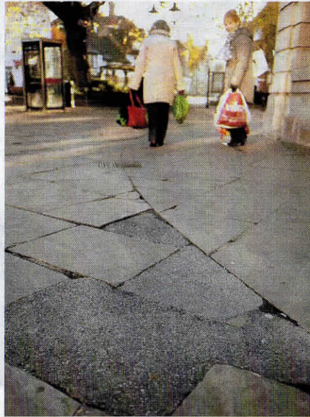
Asphalt patching in Horsham's Carfax.
