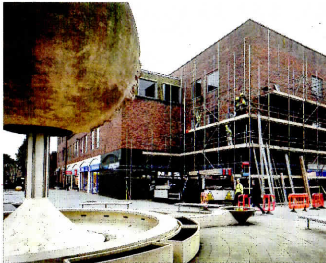
Work on Bishops Weald House in Horsham
