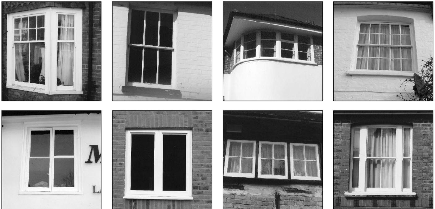
Where existing wooden painted windows are particularly good, it is always worthwhile considering secondary glazing - frameless, plain, sliding glass panels - behind the external windows. These are virtually invisible from the outside and improve insulation. Their use has proved successful on listed Georgian windows.
