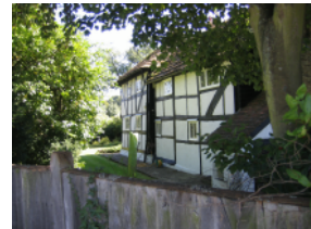
8. C15th wealden building, one of the oldest properties in Horsham.
