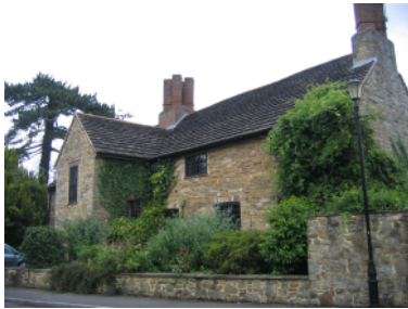
5. Unique stone built house with a Horsham stone roof. The last surviving remnant of a once fine mansion
