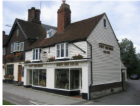
1. C17th three bay timber framed building .
