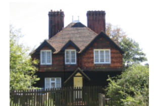
4. Pair of cottages with decorative tile hanging and ornate brickwork on the tall chimneys.
